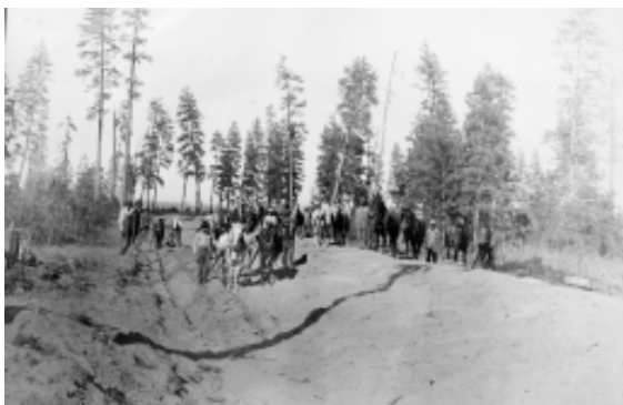
Digging an irrigation ditch with horse teams.
